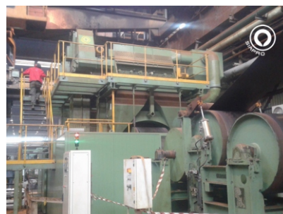
Descaling Coil Steel Strips
